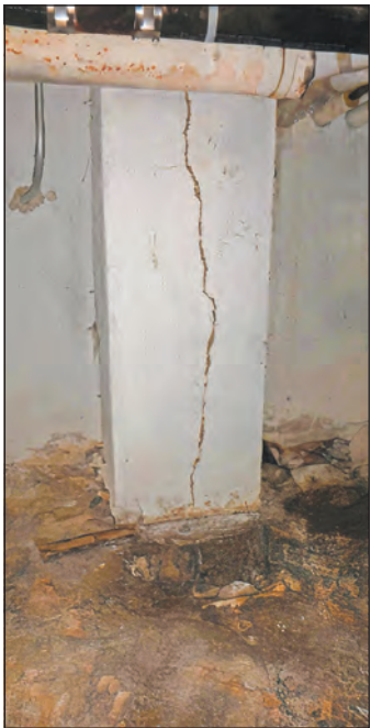
USD 259 provided photos show support pillar in basement with a large crack
