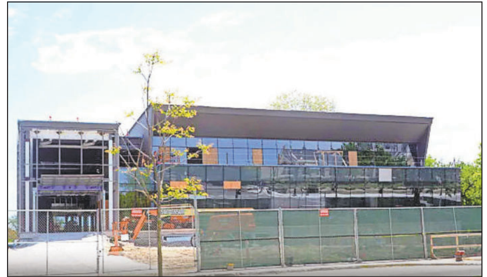
Obama Presidential Center Draws Criticism, Inspires Hope As Construction Continues.
