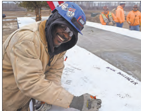
A worker adds his signature to the beam
