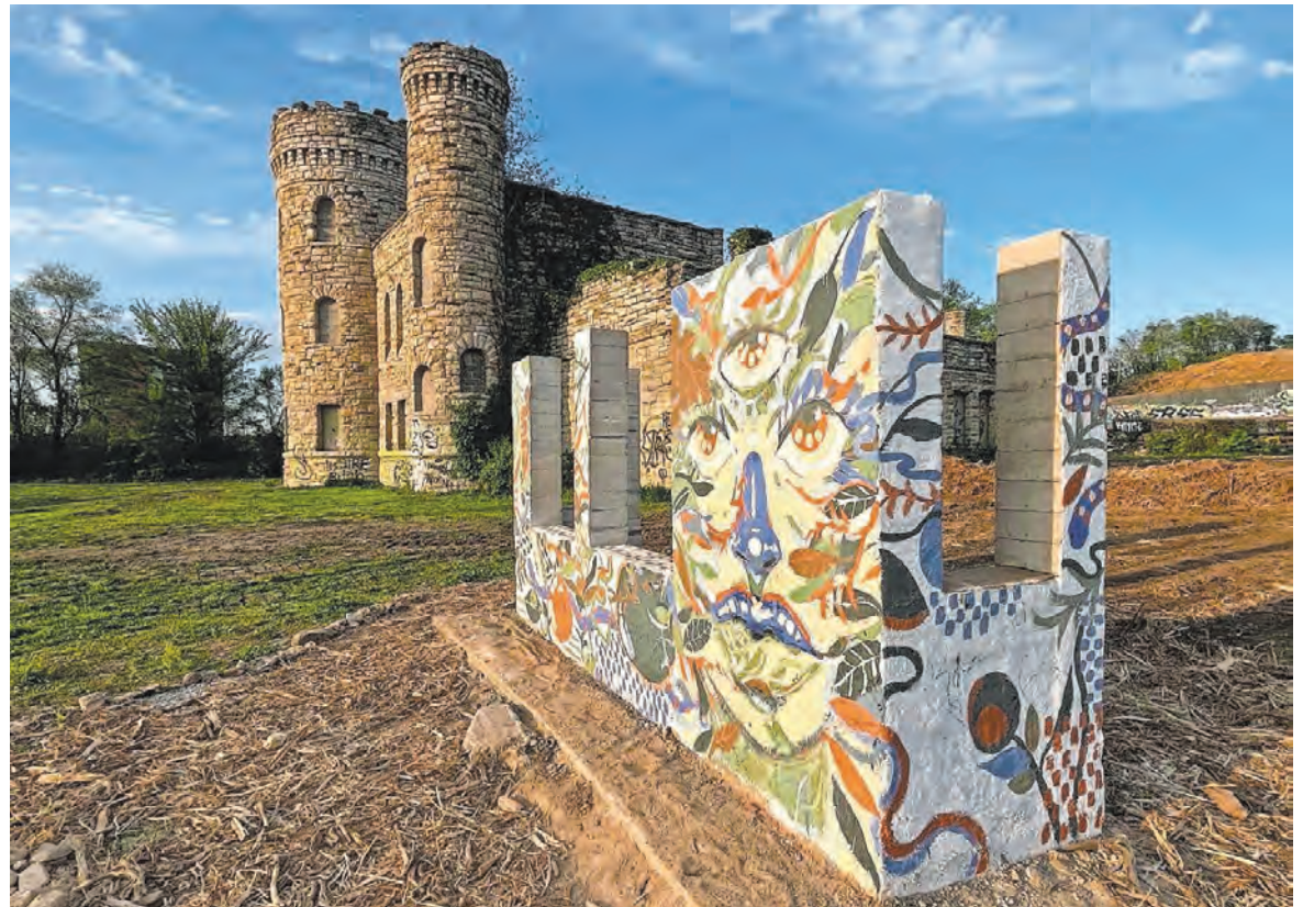
Riddle has built a proof-of-concept wall on the lot downhill from the Vine Street Castle. You can stop by and check out how a CEB house comes together.
