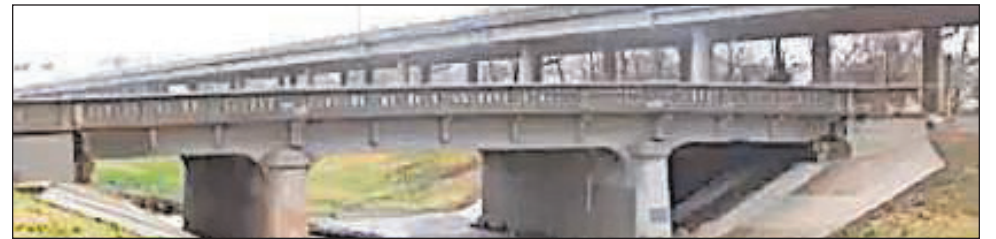
15th Street bridge to be replaced
